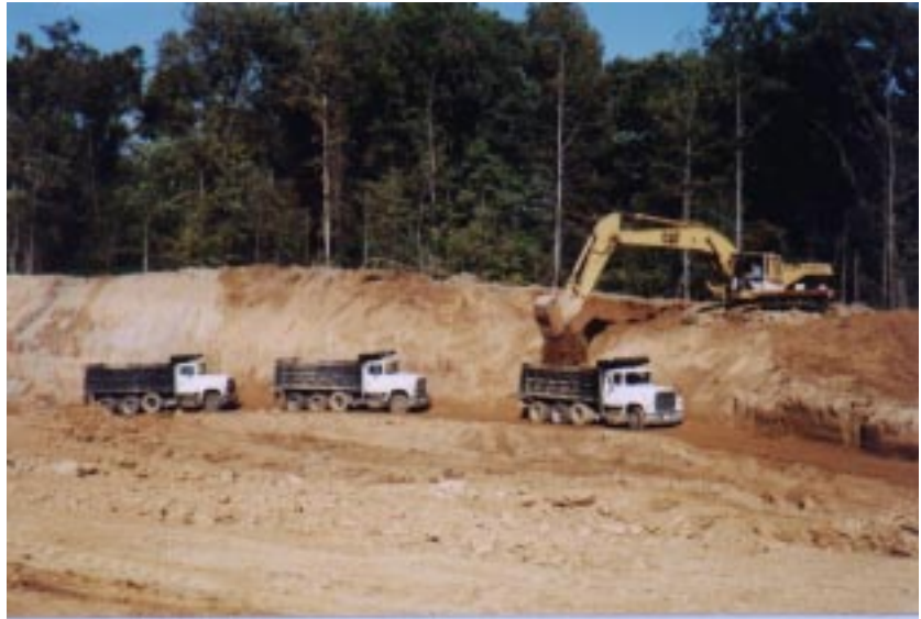
Figure 1: Hydraulic excavator loading trucks at a construction site.
