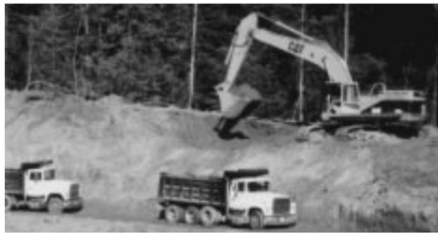
Fig. 1 Excavator loading a truck with soil in a typical mass excavation work scenario
